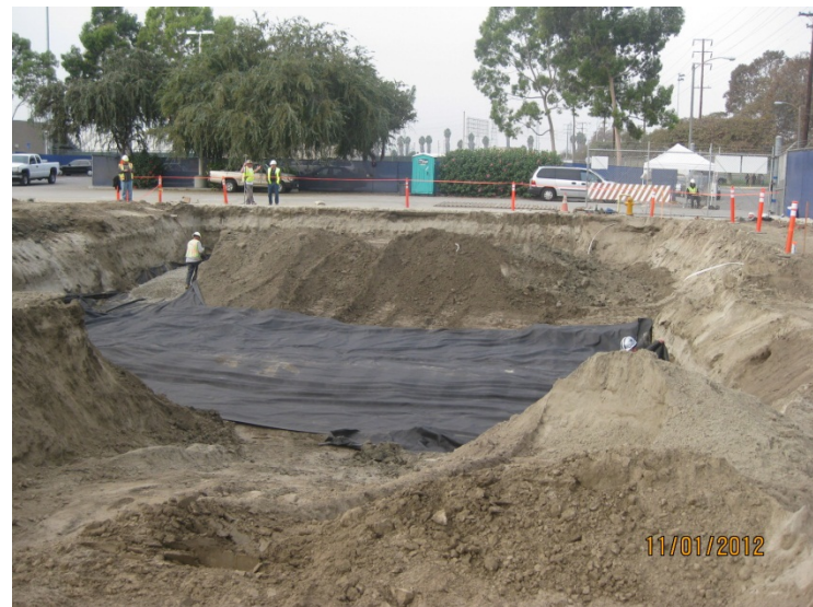
Laying Rock and Fabric Building 300
