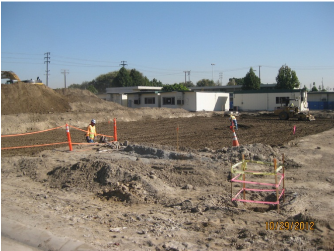
Soil Stabilization of Building 100 Complete
