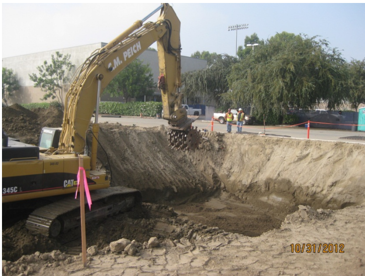
Excavation and Stabilization of Building 300
