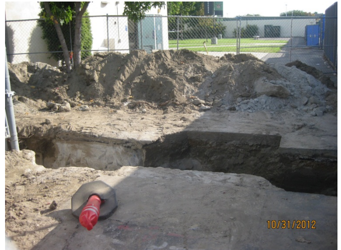
New Electrical Service Continues Trenching
